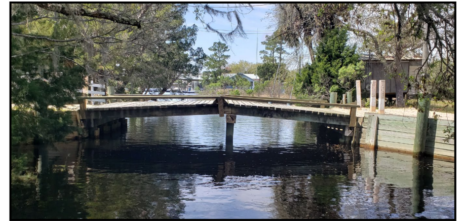
Existing Granger Drive Bridge
